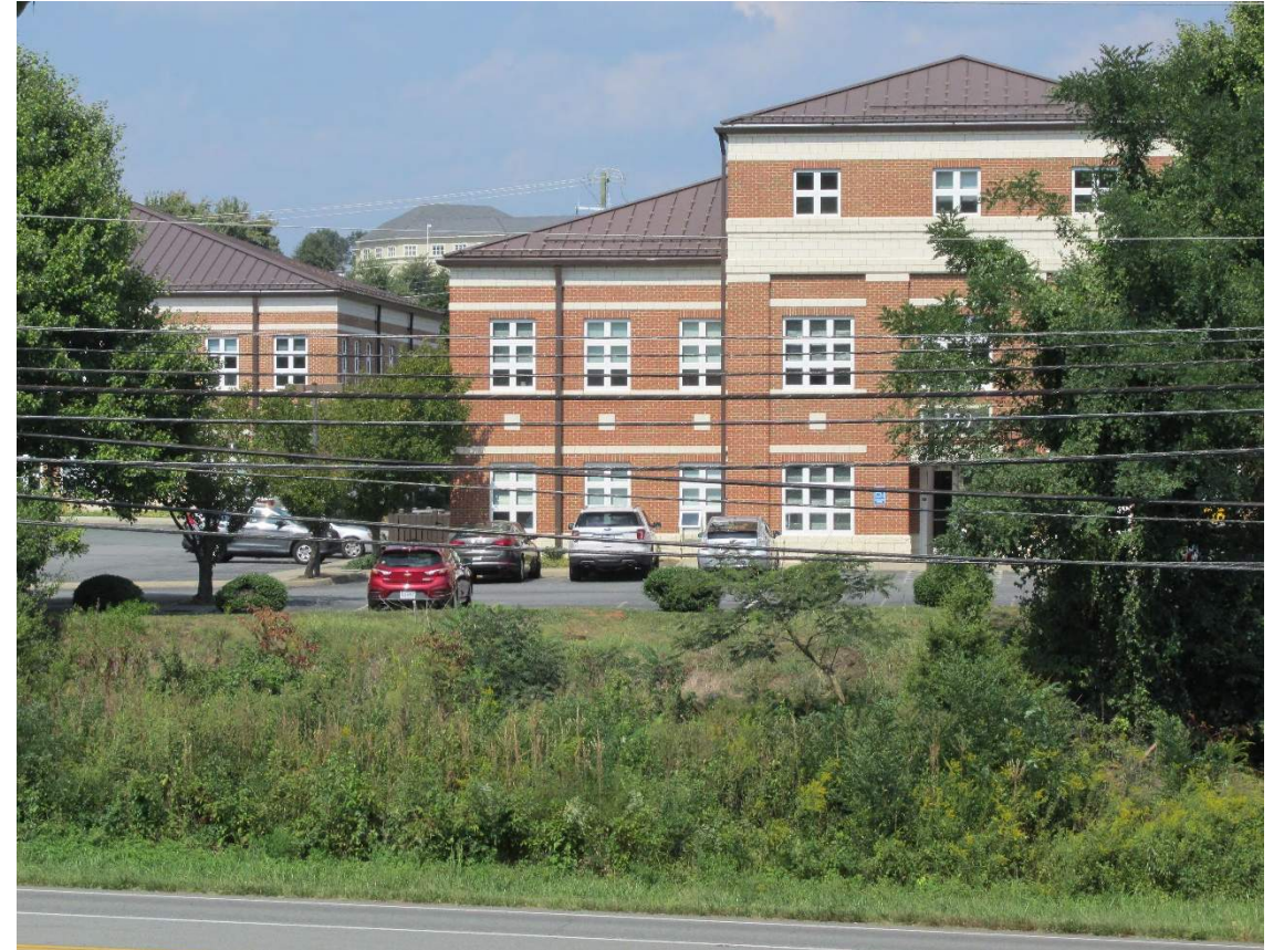
Figure 9: Existing commercial buildings to the north, on Old Ivy Road.
