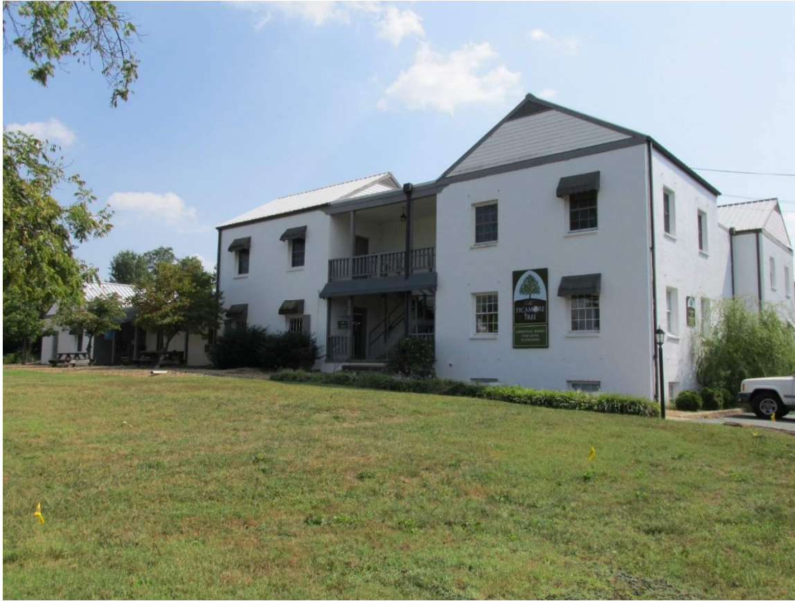
Figure 4: The existing commercial building.
